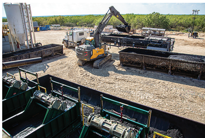
Fig. 4. Reclaiming as much fluid as possible from downhole cuttings is the goal of a solids-control system. Here dry cuttings are loaded for haul-off and disposal.
