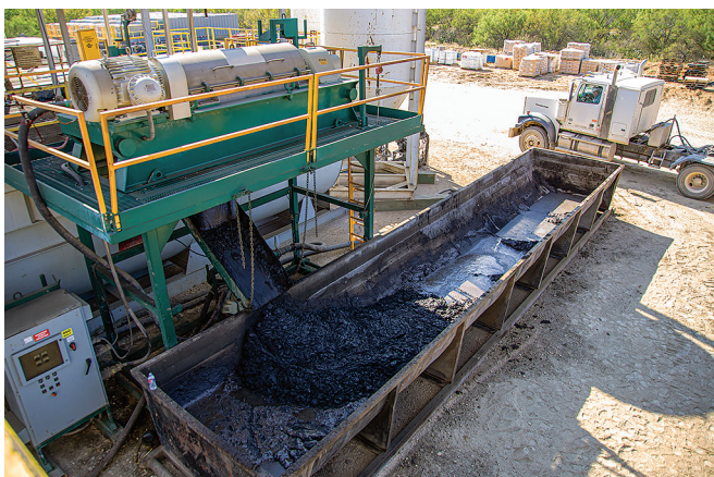
Fig. 3. A key component of the solids control process is the centrifuge, which removes fine particles from the mud.
